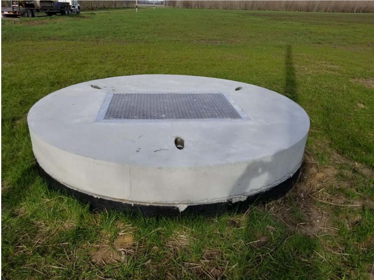
The newly mounted pit top with differently positioned pit hatch.
