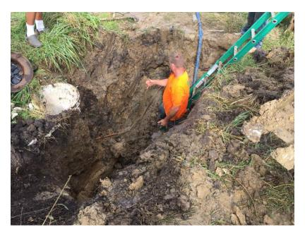
Brine Tank #1 was cleaned on October 5, 2016 by Bodine Environmental of Decatur. The material removed from the tank is disposed of at Waste Management. Pictures below are the lateral lines that were cleaned and the sand on the ground that was in the laterals.
