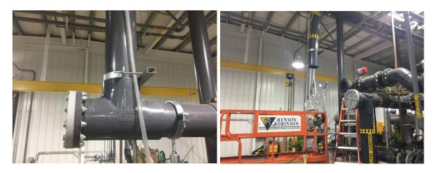
**Well 8 Pump Replacement.** Brotcke Well and Pump was on-site in early November to perform rehabilitation work on Well 8. After treatment, Brotcke recommended replacement of the pump. A replacement pump belonging to SSWC was on-site and was used to replace the pump. Well 8 was placed back in service on November 22, 2017.
