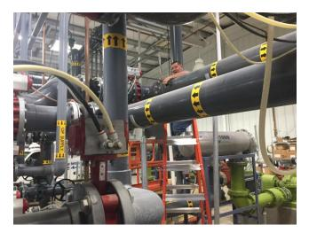
Leak on the Backwash Line #1. A leak was found on Backwash Line #1 early in the morning of September 10, 2017. Henson Robinson was contacted to secure the parts necessary and make repairs. Repairs were made on September 14, 2017. The line can be isolated and the plant can operate on one backwash pump so there was no interruption in service. Pictured below on the left is the elbow that was leaking and the replaced elbow is pictured on the right.
