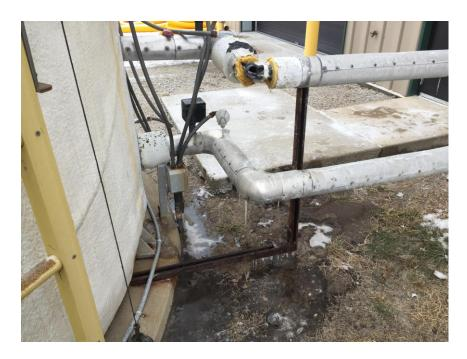
**Sodium Permanganate Line Freeze.** On January 2, 2018, the Sodium Permanganate line started to freeze from the extremely cold temperatures on January 1, 2018. Pictured below is a small cover constructed by Plant Operations staff. The line was thawed using a heat gun. We then insulated the conduit and the outside of the box to help protect the line.
