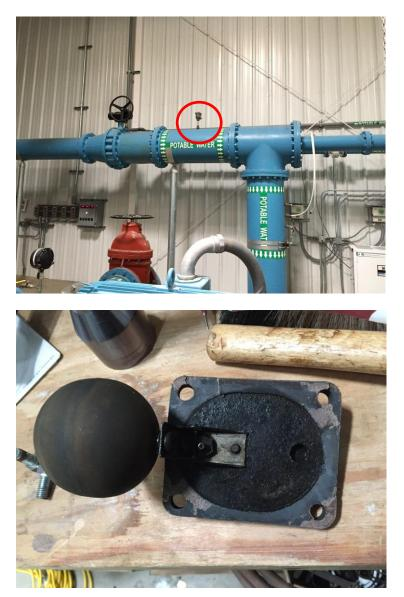
The valve was disassembled, cleaned and reassembled and placed back in service. There was no disruption in service.
