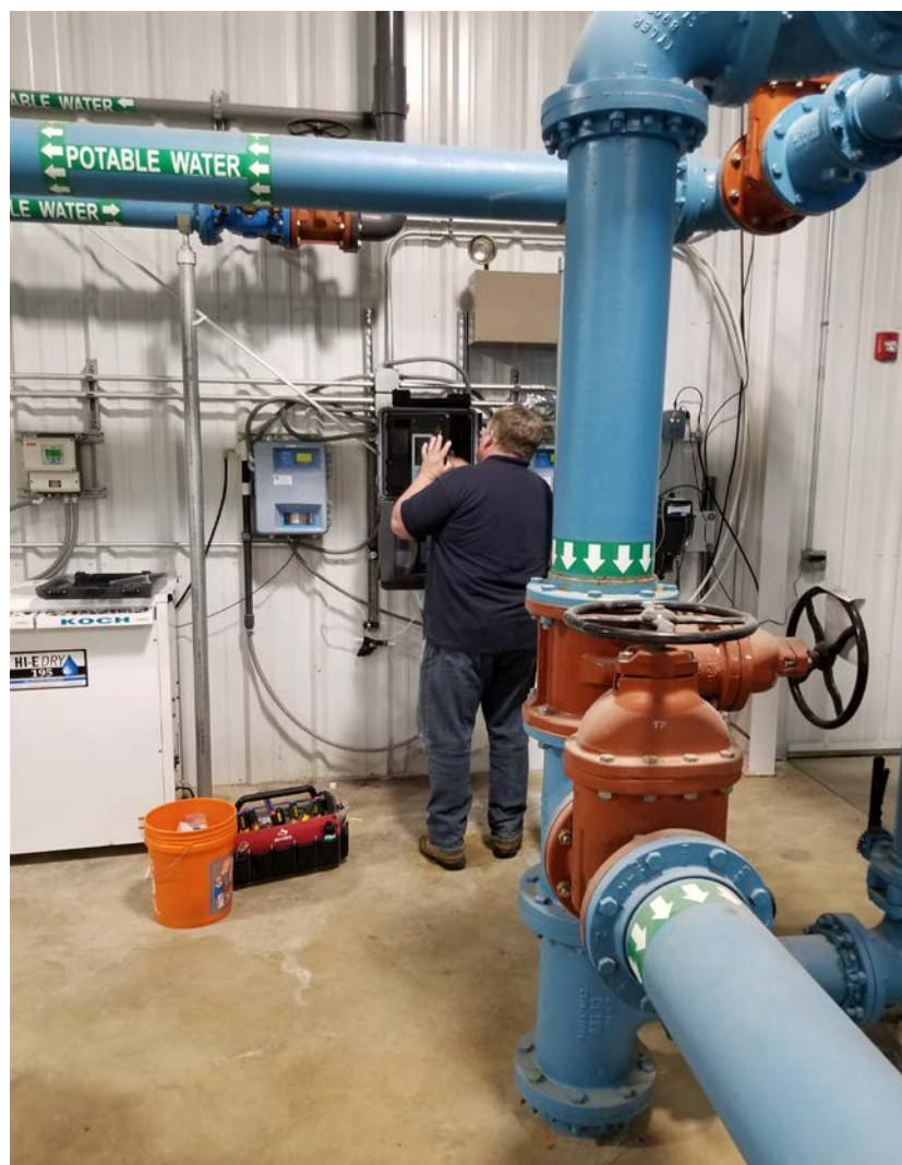
Eric from hach programming and performing start up procedure on the Hach sc5500 monochloramine analyzer
