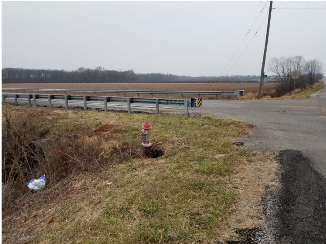
Hydrant at Mansion Rd and Curran Rd was damaged, causing a leak.
