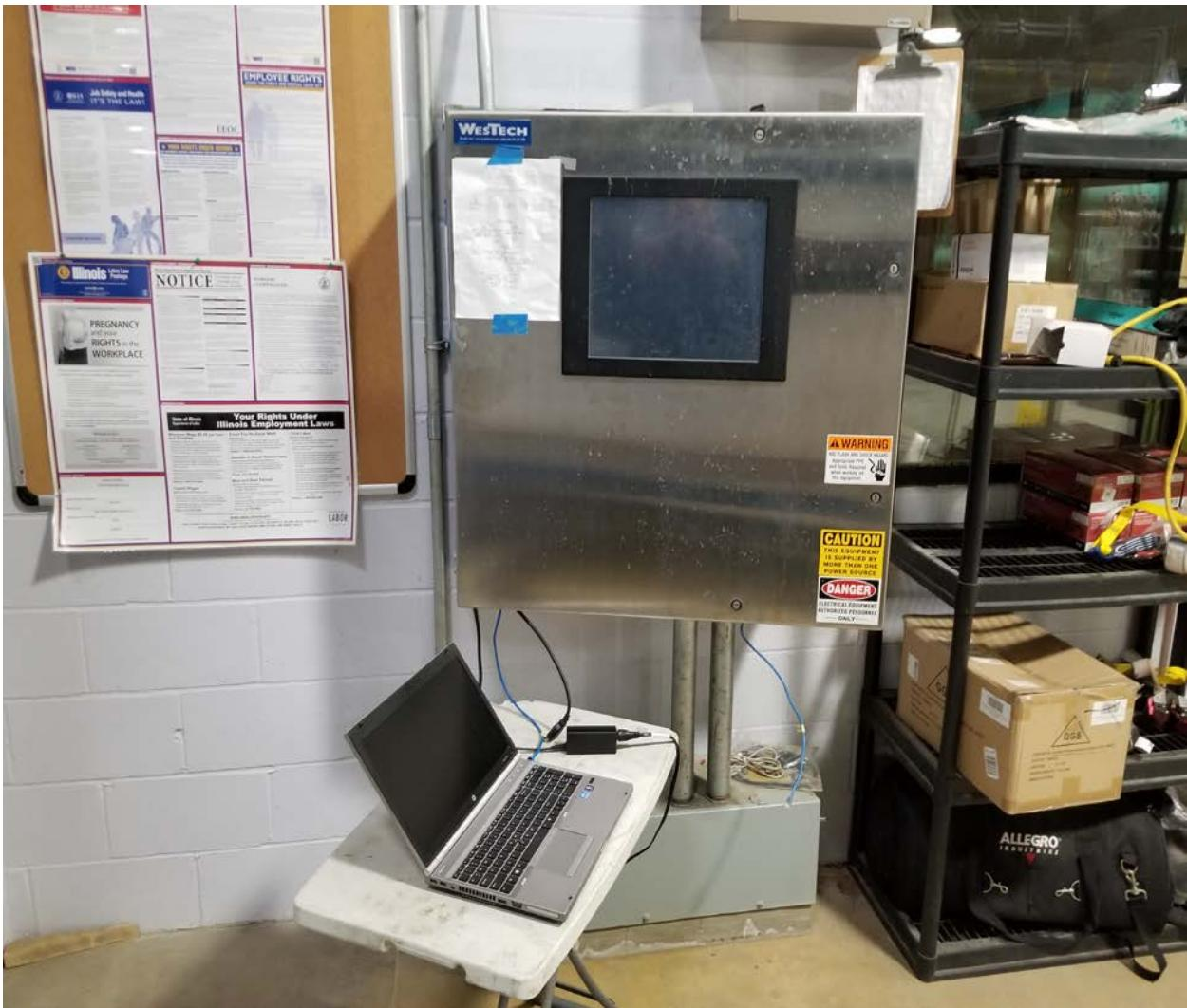
Installed backup computer to monitor and control UltraFilter control PLC.
