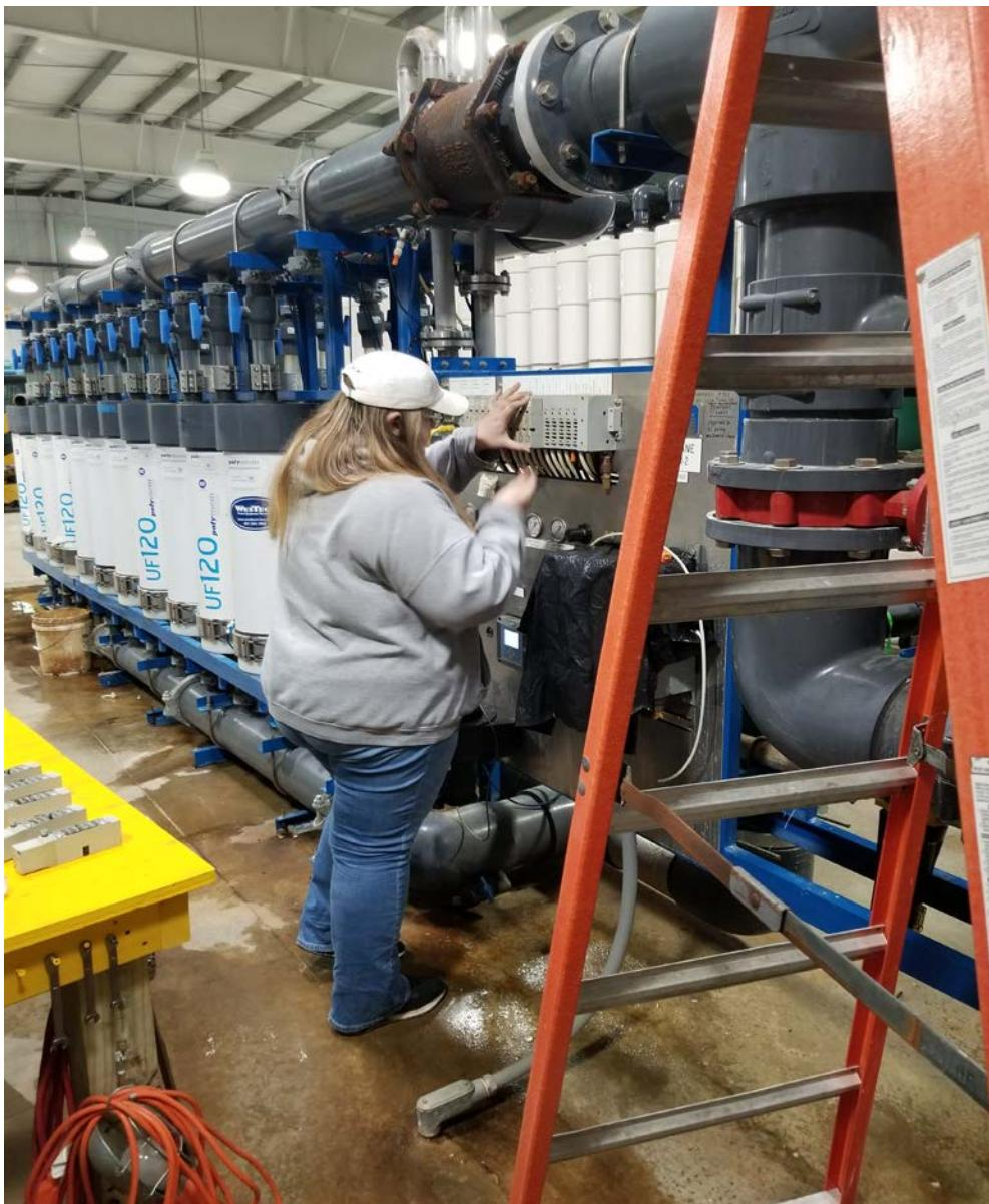
Assistant Operator Katie Krall reinstalling the air valves that trigger the actuators after purging the system of water and cleaning out the manifold.
