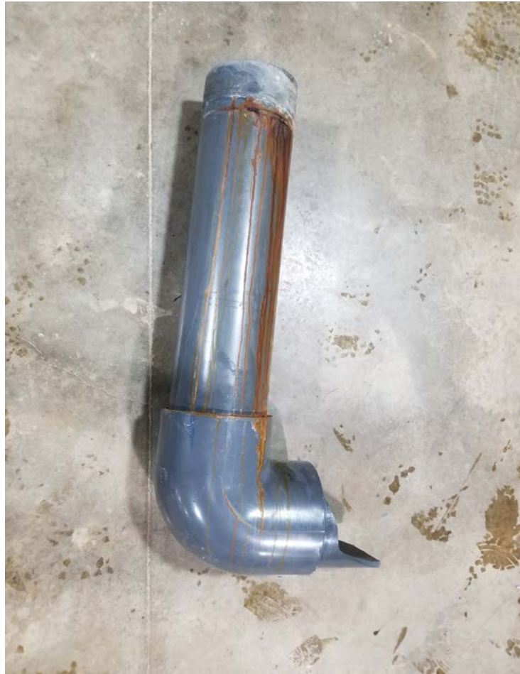
This is the section of line that came apart and broke off in the Chloride waste discharge system.
