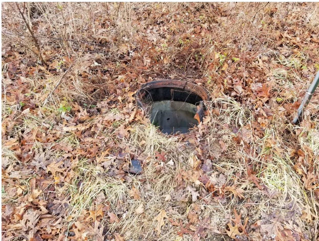
Air purge valve ring had been damaged and the pit lid is missing.
