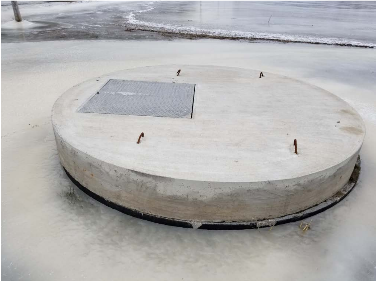
Current pigging station pit lid that is slated to be replaced.
