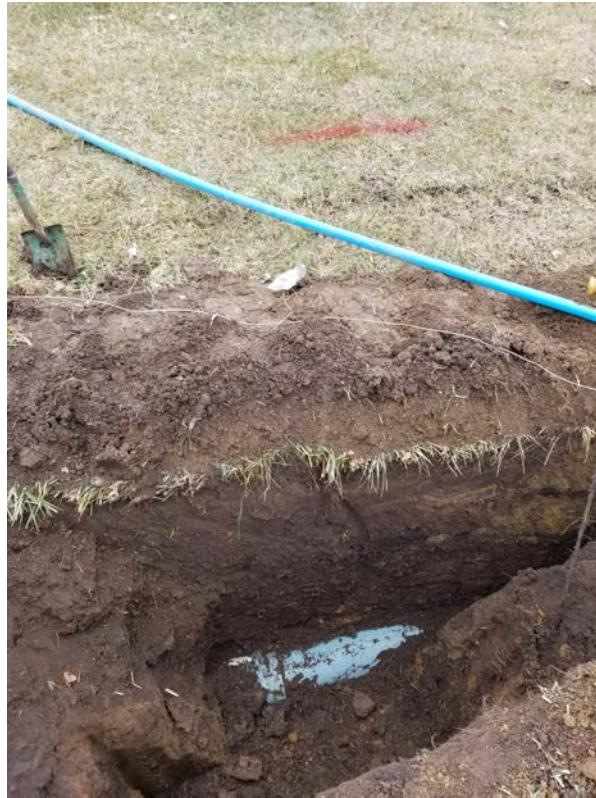
While running the service line to our new customer the contractor discovered SSWCs waste effluent line. This line had not been located by USIC. USIC was called and it was then properly located.
