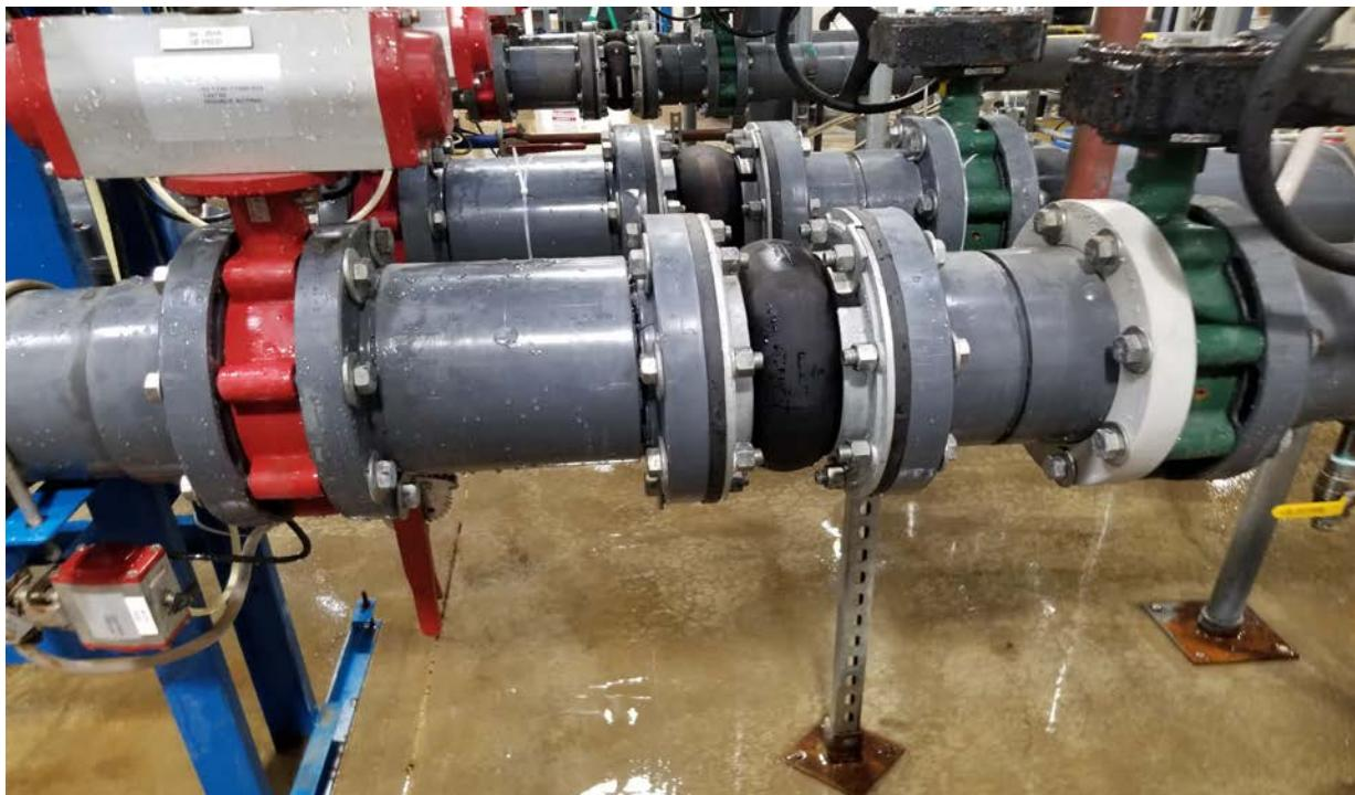
On January 6<sup>th</sup> AAC arrived on site at SSWC to program for the New Berlin booster station. While adding the new program, AAC caused the Ultrafilter program to malfunction. This malfunction caused the LSPs to ramp up to max speed. This in turn caused a pressure surge that shut train 1 and 3 to shut down. It also caused damage to train 2. Some of the damage is this flange that burst.
