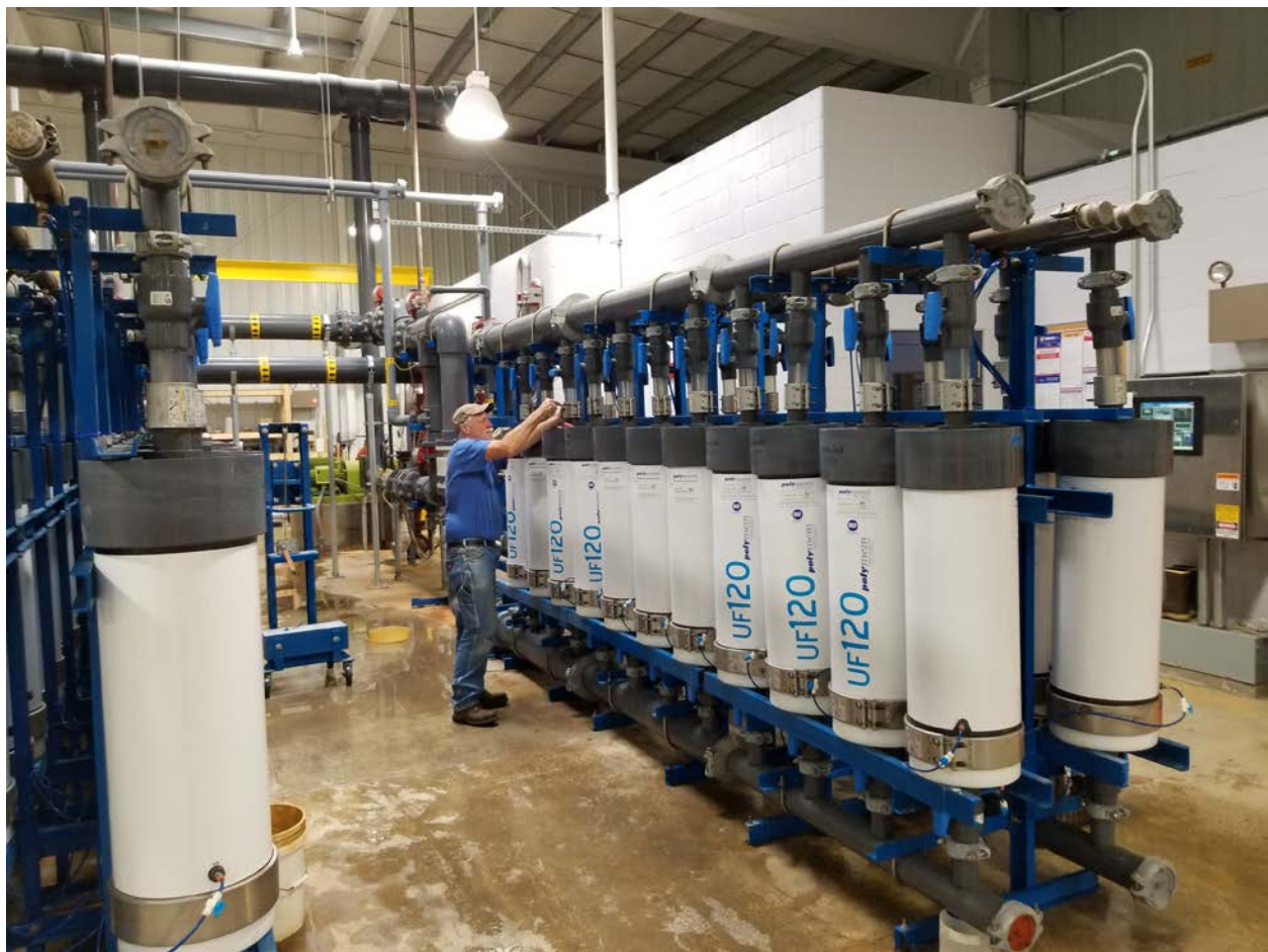
Operator Kevin Canham installing the filter cartridges from filter train #1 onto filter train # 3
