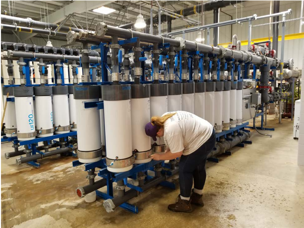
Assitant Operator Katie Krall removing an old filter cartridge from train # 3
