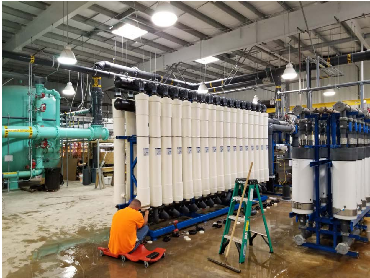
July 24 th - 26 th , new rack for Toray filters was installed.
