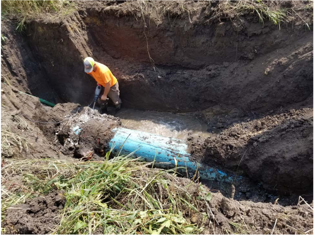
Contractor Loellke removing over flow concrete from the thrust block on the raw water line to gain access to the butterfly valve for removal
