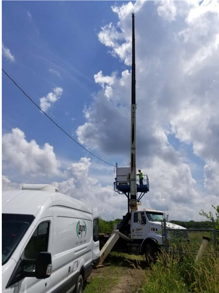
Layne pulling well#7 to begin the treatment process.
