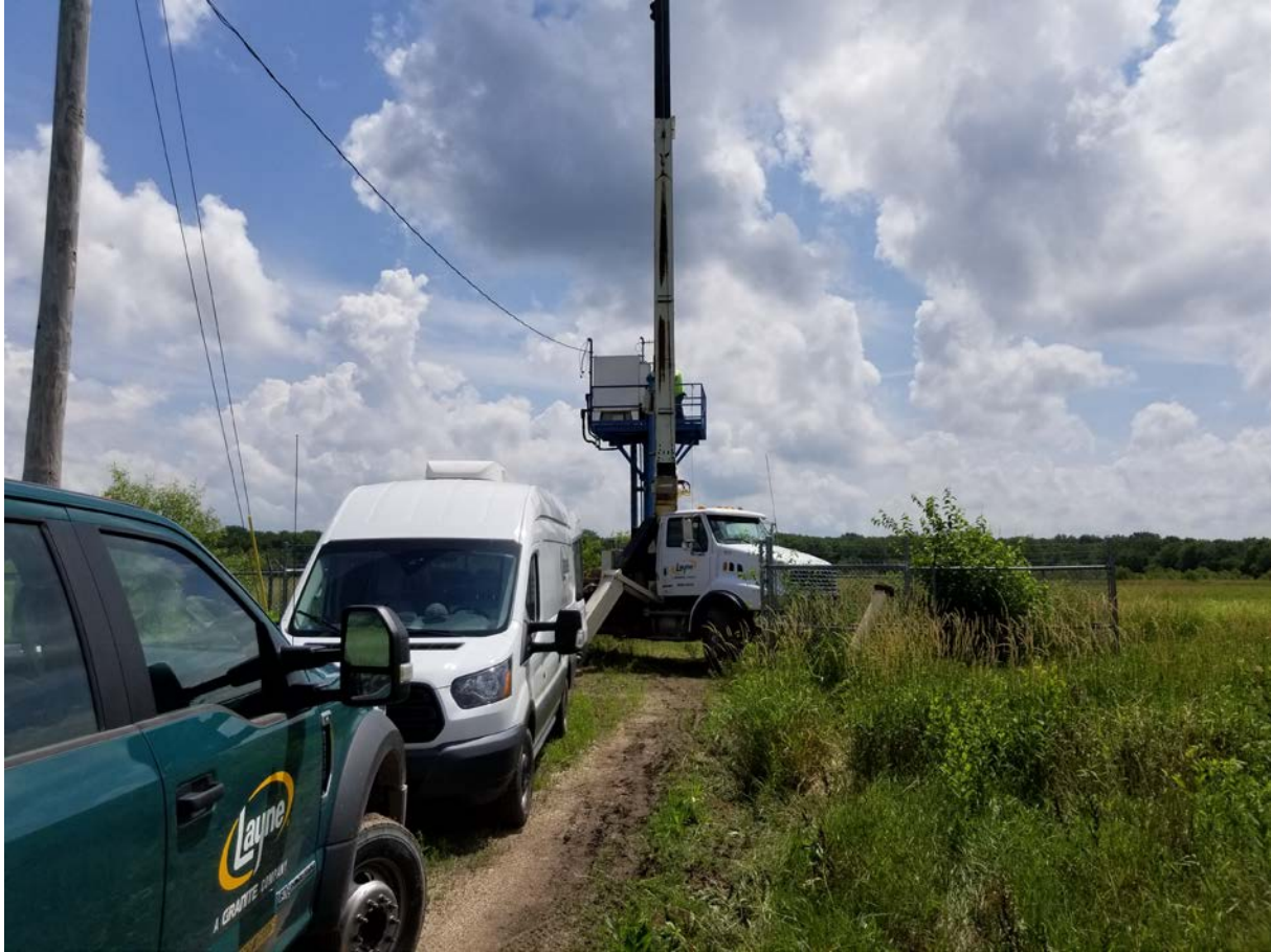
With the sonic cleaning complete, Layne is setting up to take video inspection of the well.
