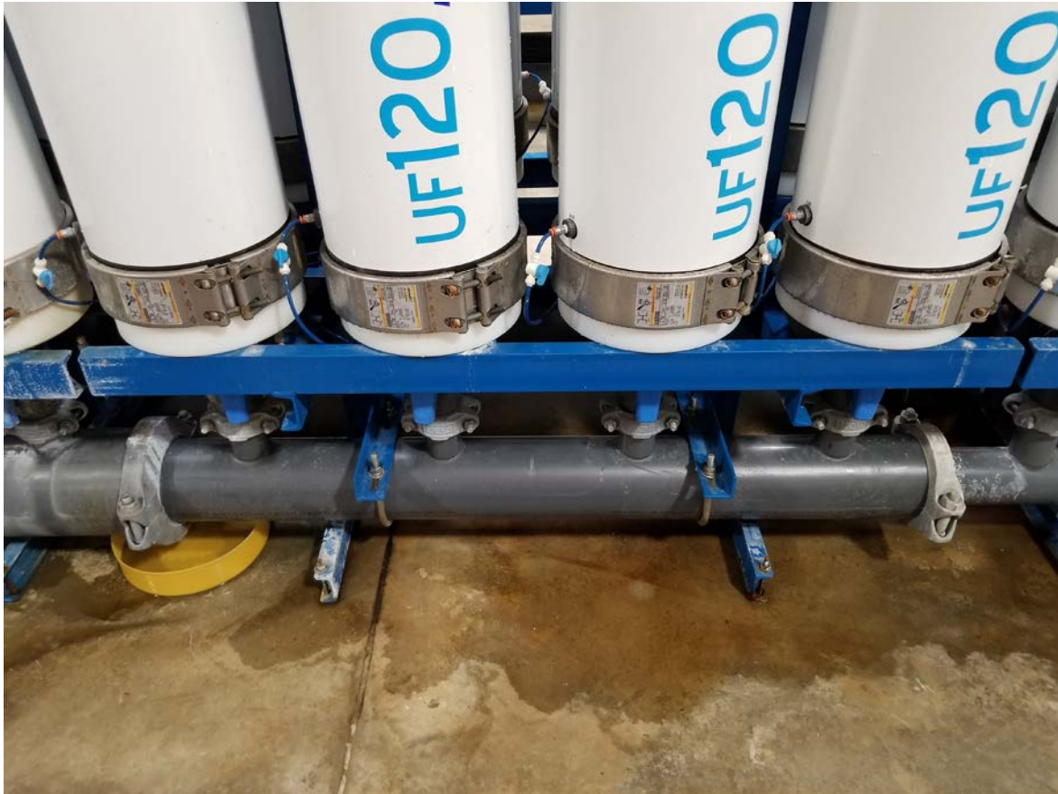
Newly installed center manifold on train #2
