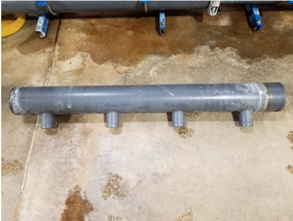
Freshly uninstalled middle manifold from train #2. Manifold had been leaking for around the groove lock.
