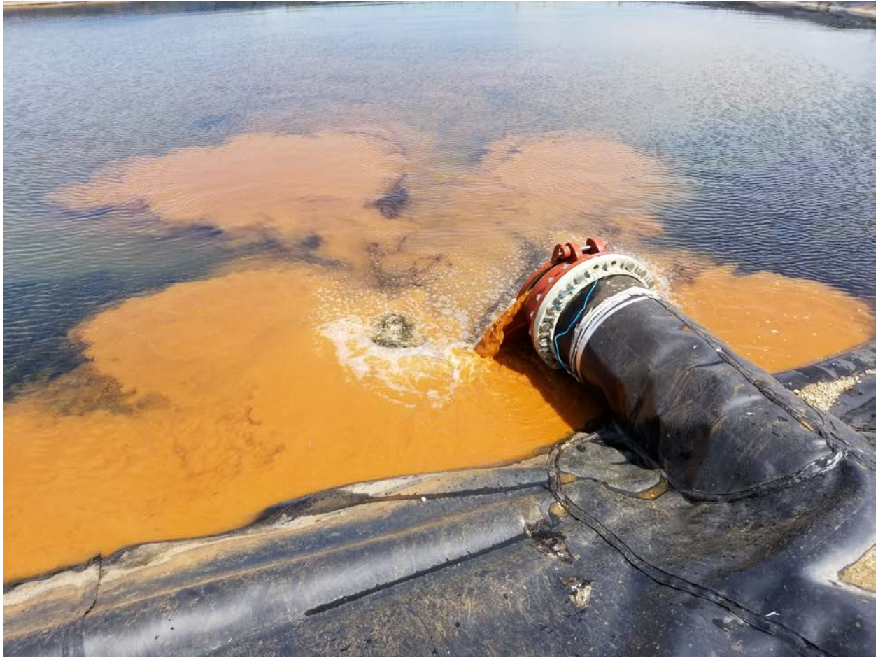
Flushing iron from the raw water line.
