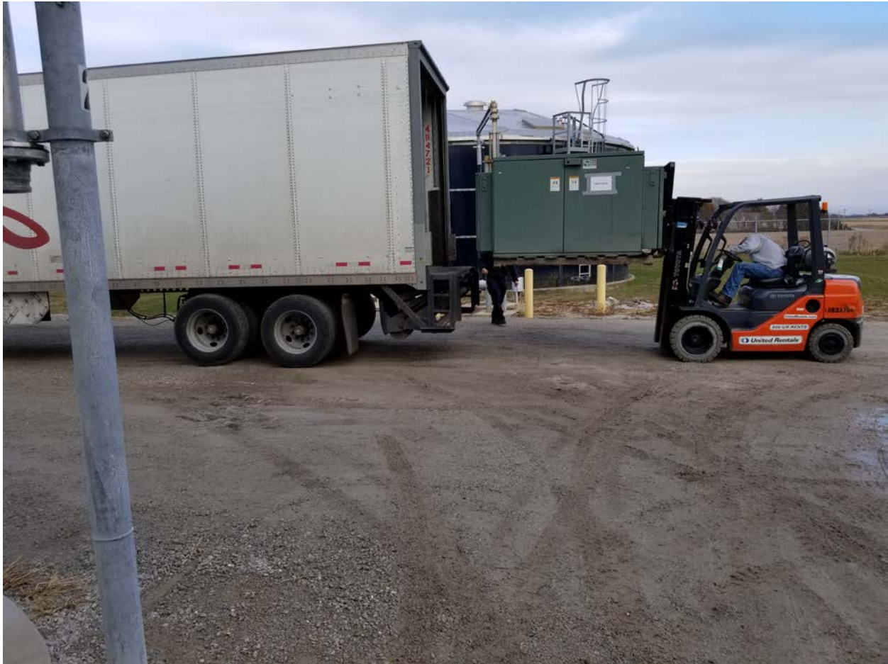
Kevin Canham loading transfer switch for delivery to S&C Electric for inspection.
