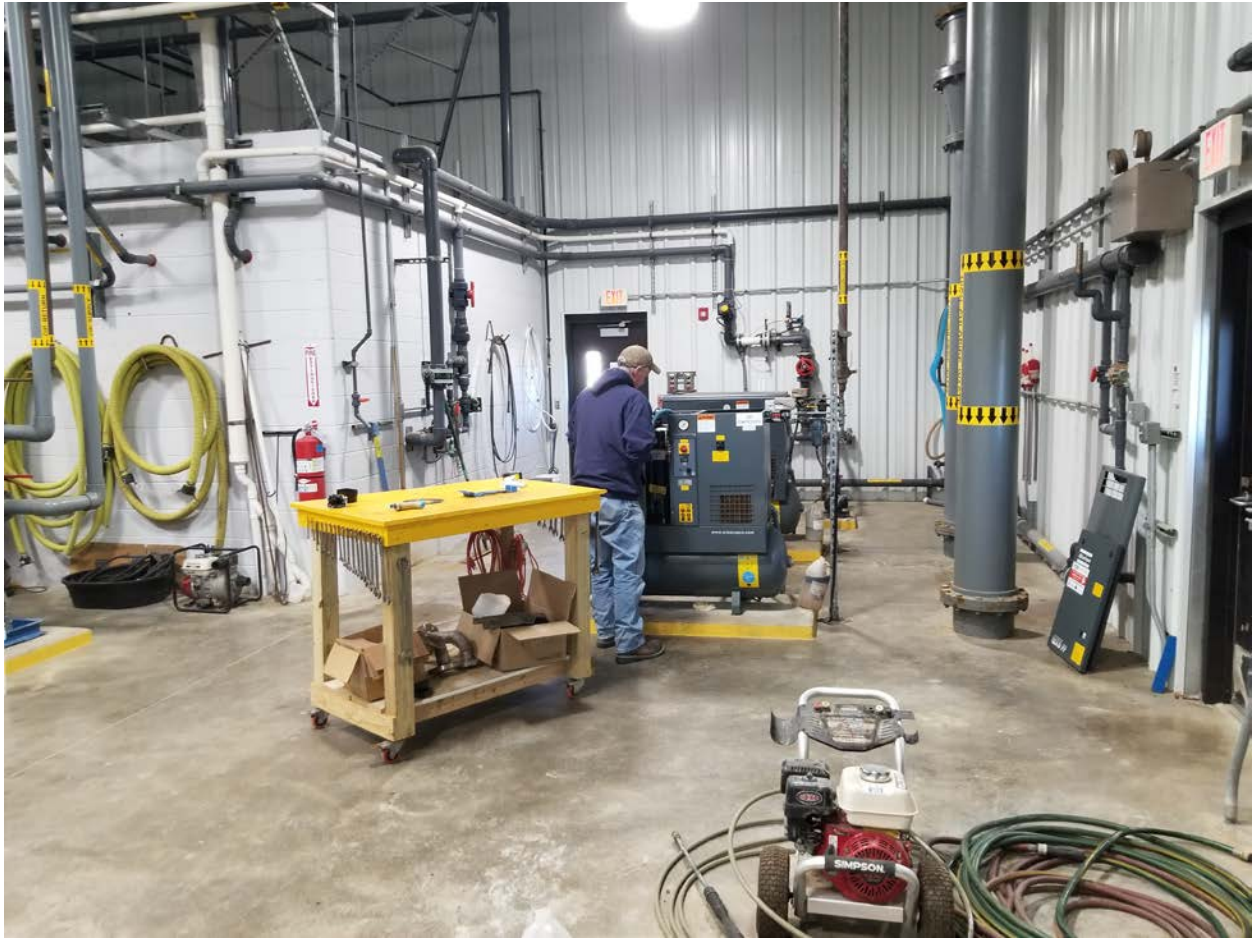
Operator Kevin Canham replacing a pressure switch on compressor #2
