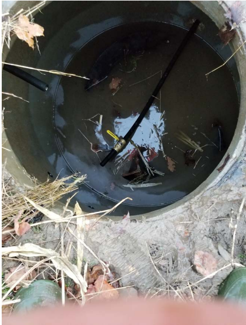
The air valve was removed and a ball valve was installed to stop the flow of water.
