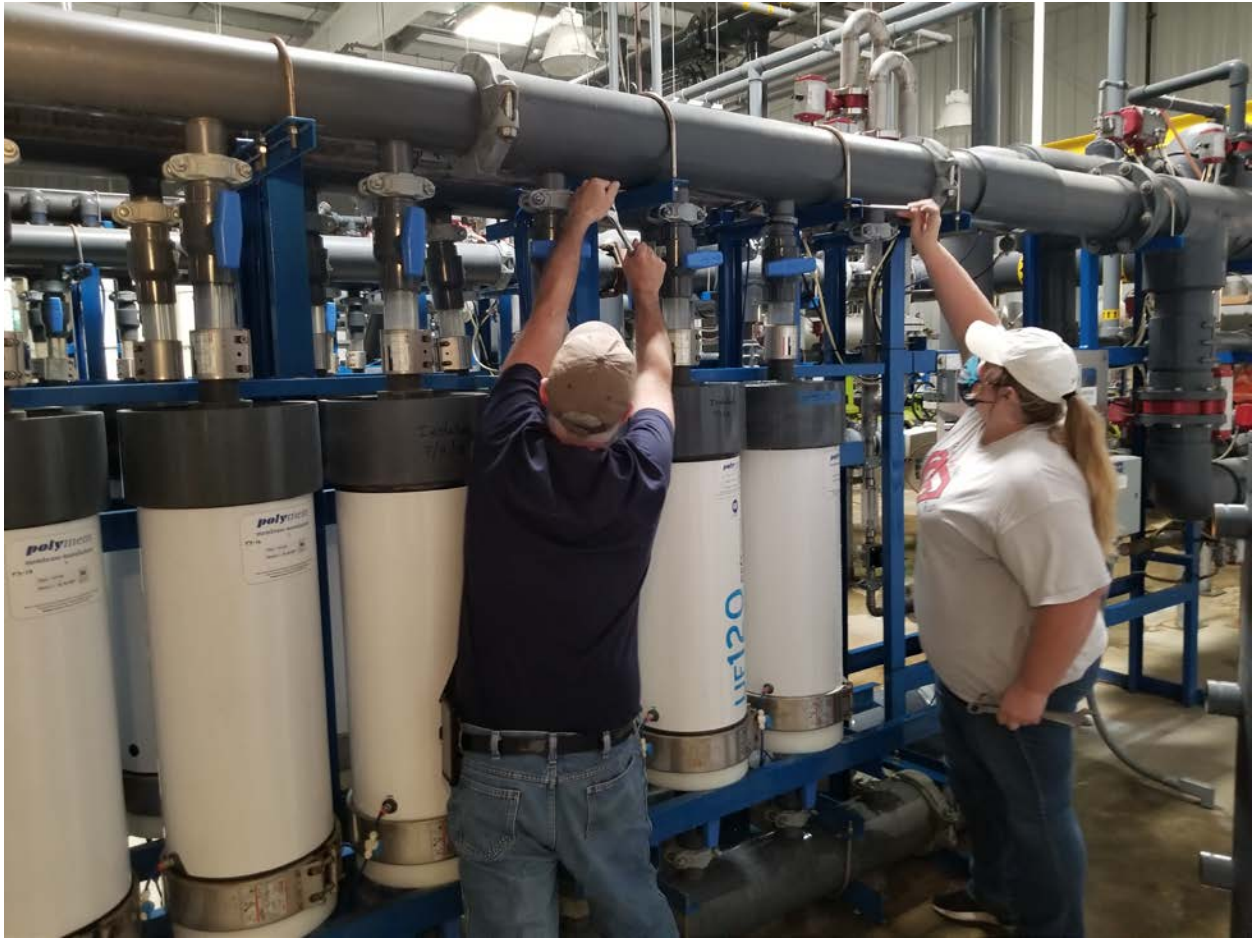
Operators Kevin Canham and Katie Krall replacing an upper manifold on train #3 that was leaking
