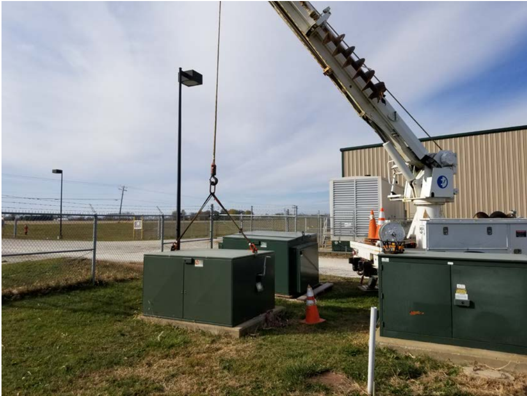
Egizzi removing the manual transfer switch and replaced it with the automatic switch
