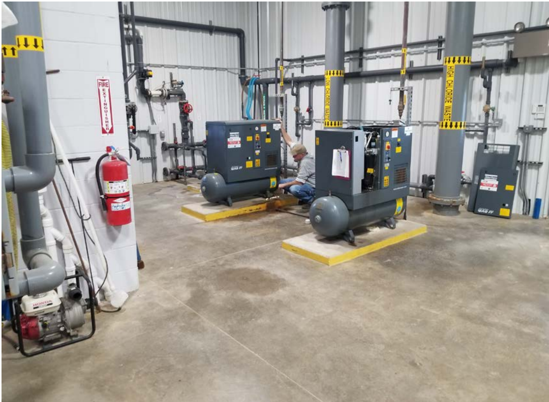
Operator Kevin Canham draining the condensate from the 2 operation air compressors. The compressors provide air to the valve system allowing them to operate. The tanks are drained on a daily basis.
