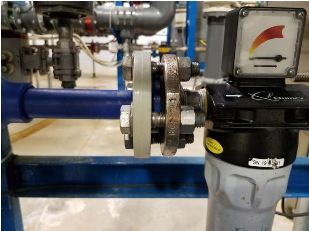
On September 2, SSWC personnel received a low air pressure alarm. Upon returning to the plant it was discovered that the bolts on the flange that feed air to the air scour system had loosened. This allowed the gasket to push out under pressure.
