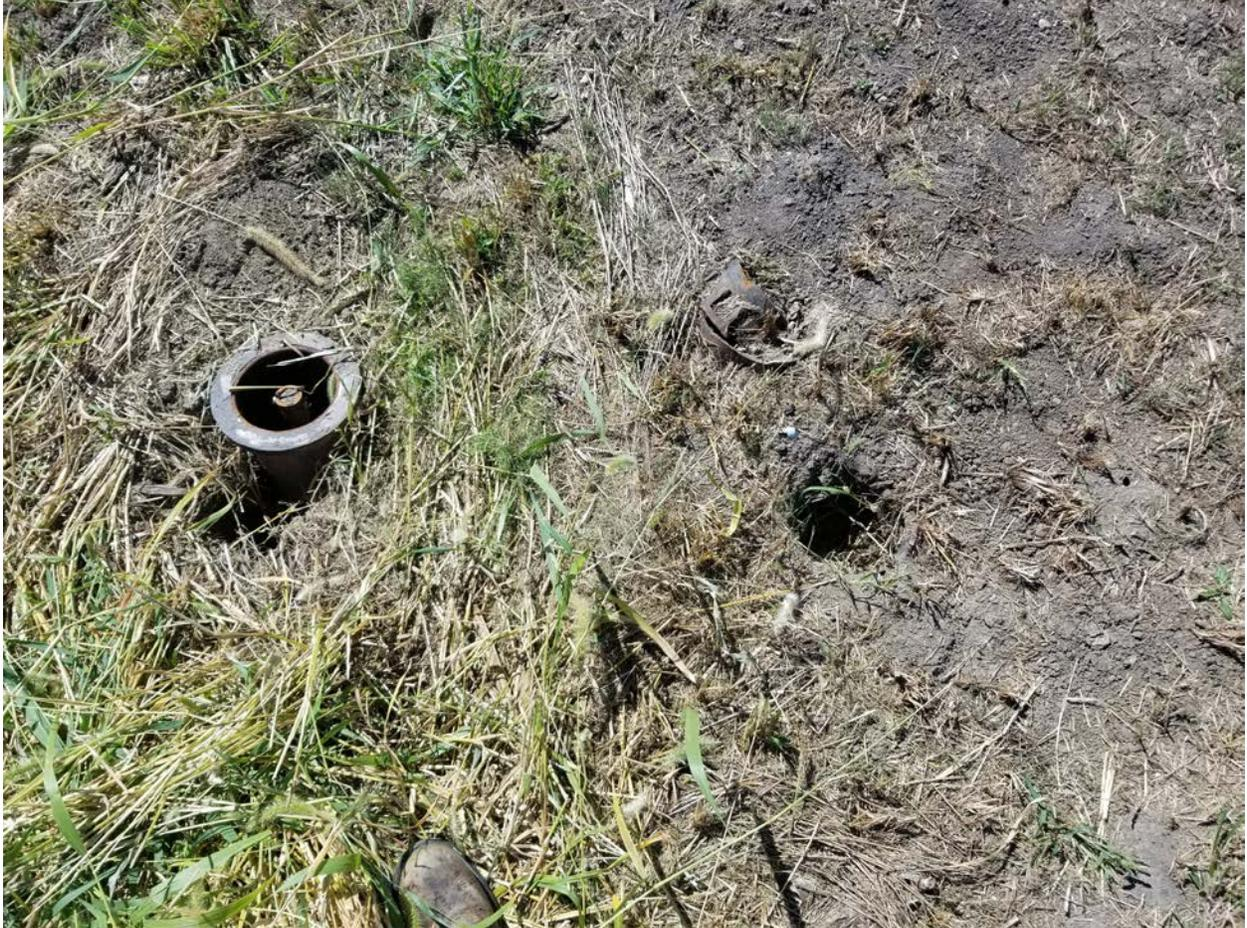
Upon closer inspection it was found that the valve box is also damaged.
