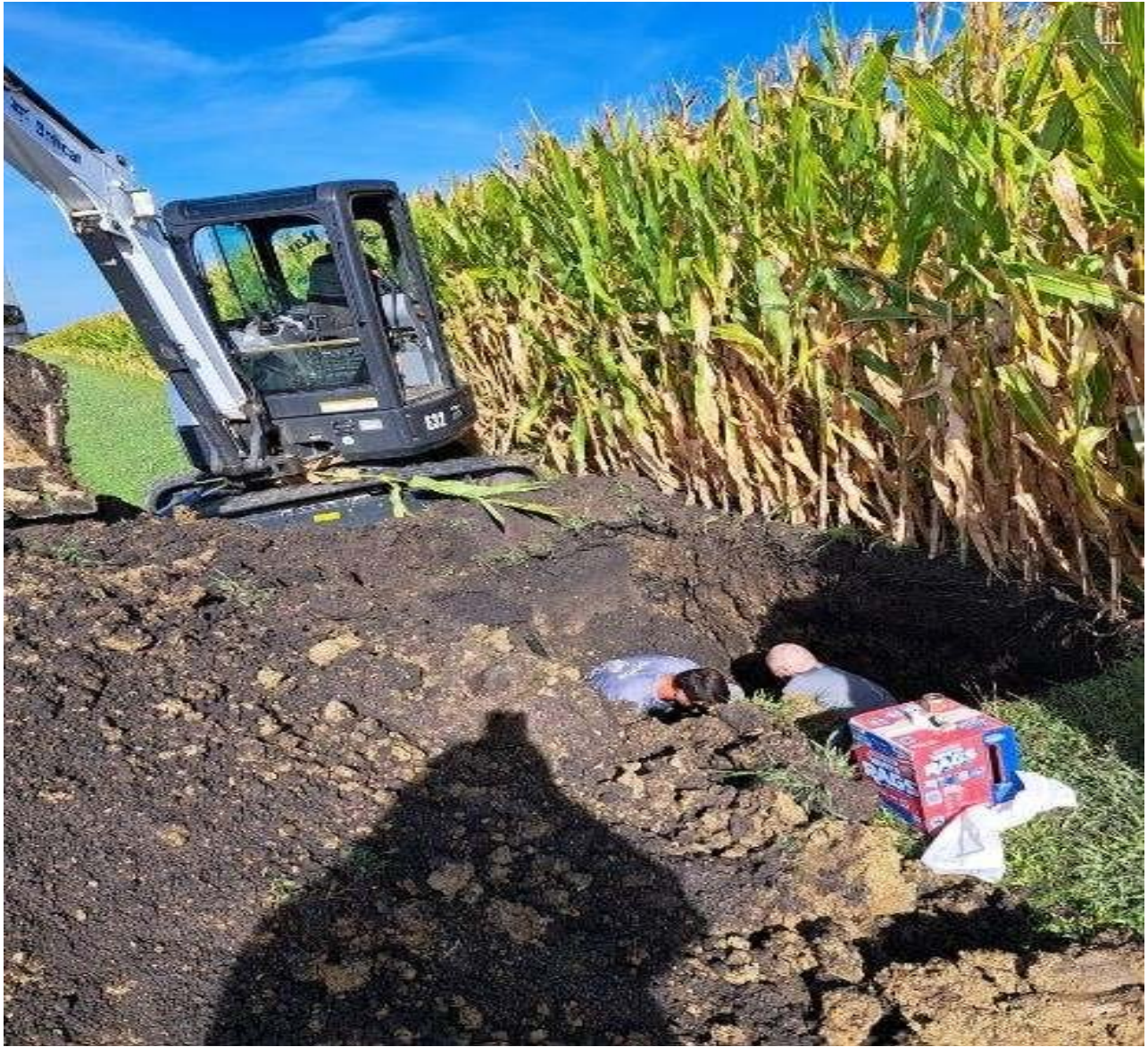
The plumbers from Steve Ray tapping the Mansion Road water main.
