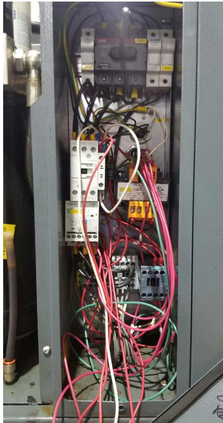
New motor start and control module have arrived and have been installed.
