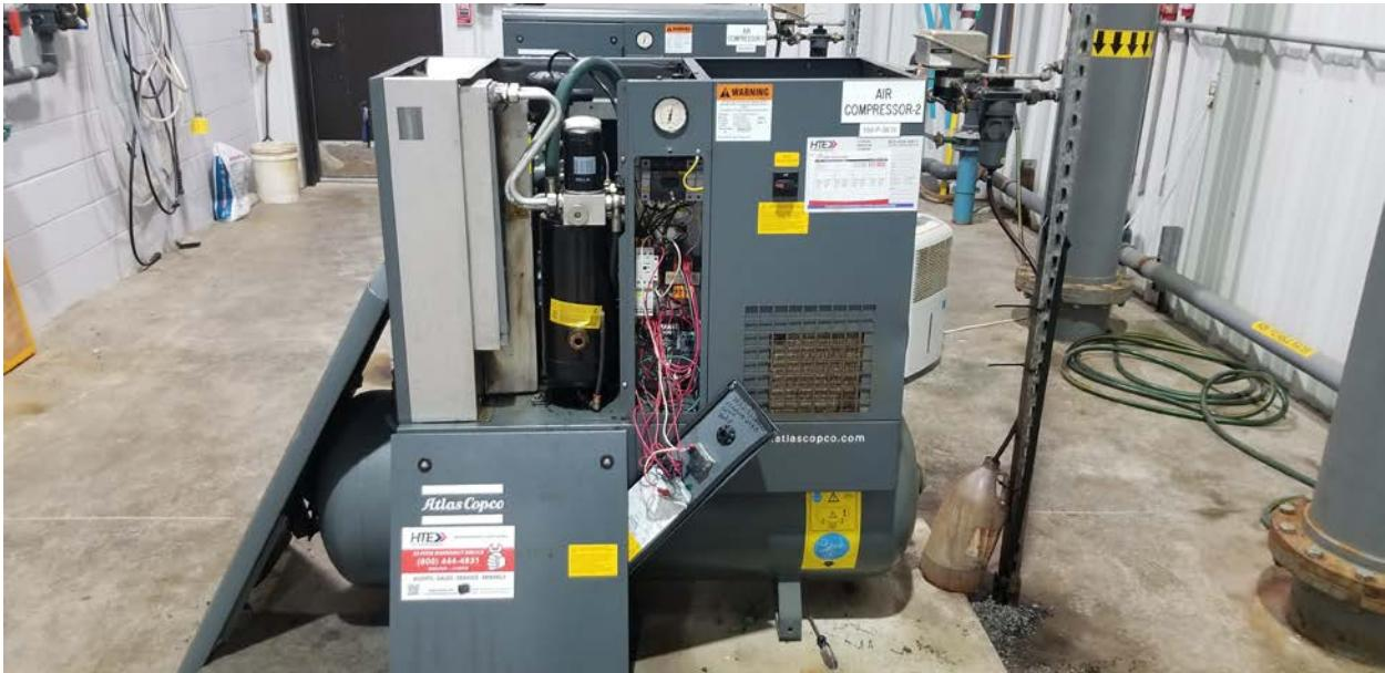
After inspection it was found that the motor starter and the compressor control module had both went bad. Parts were ordered. The compressor is also blowing oil and has been for sometime. Option are being explored.
