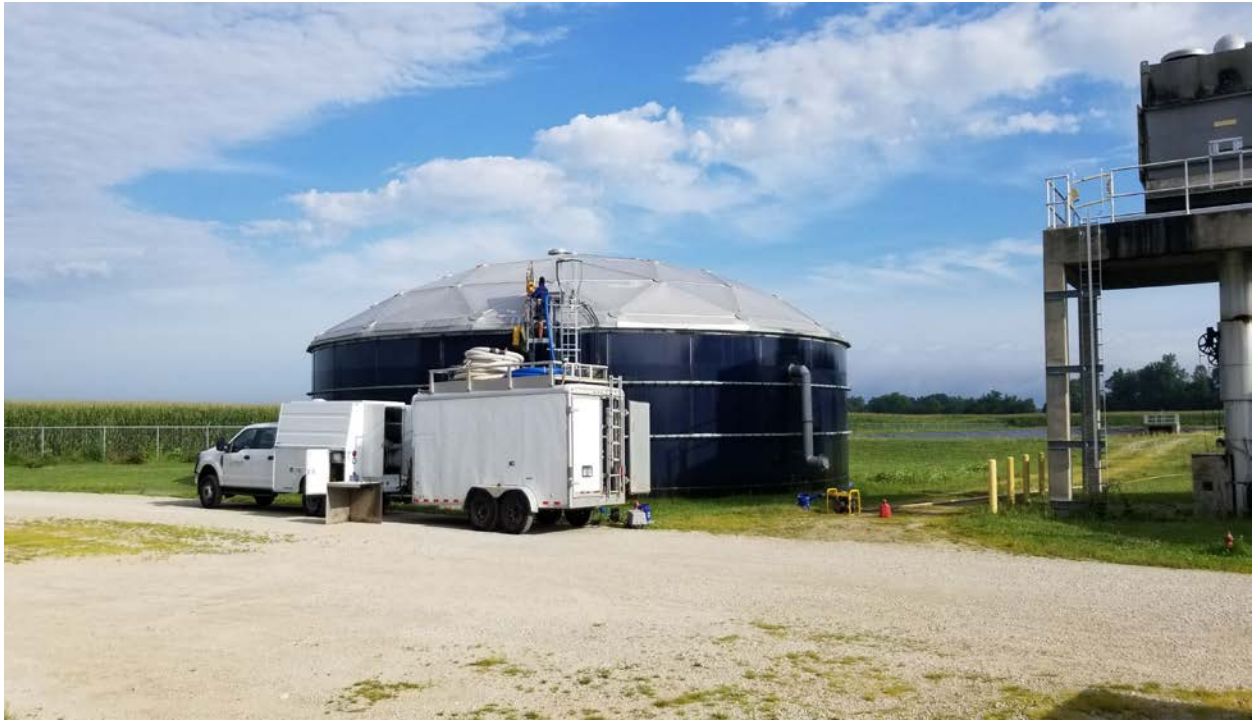
Liquid Engineering was on site to clean and inspect tanks at the plant.
