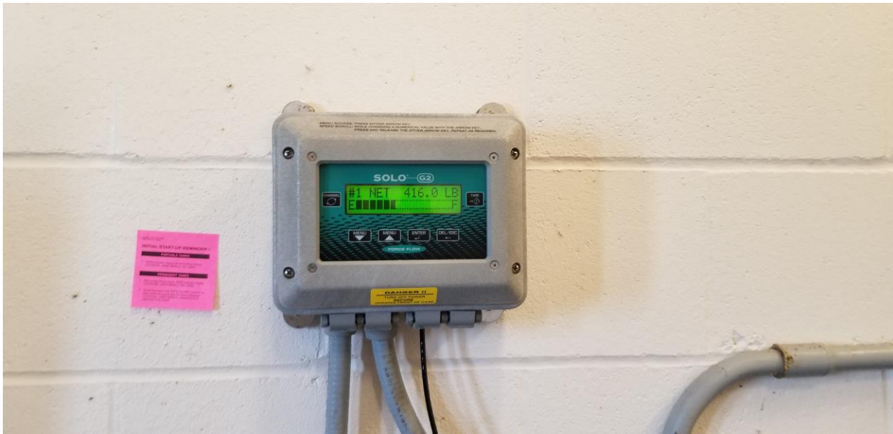
Replaced Permanganate scale and redout.
