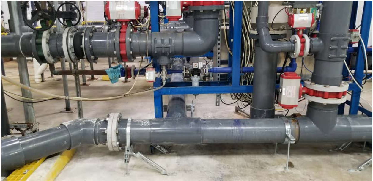
New drain connection for train #2
