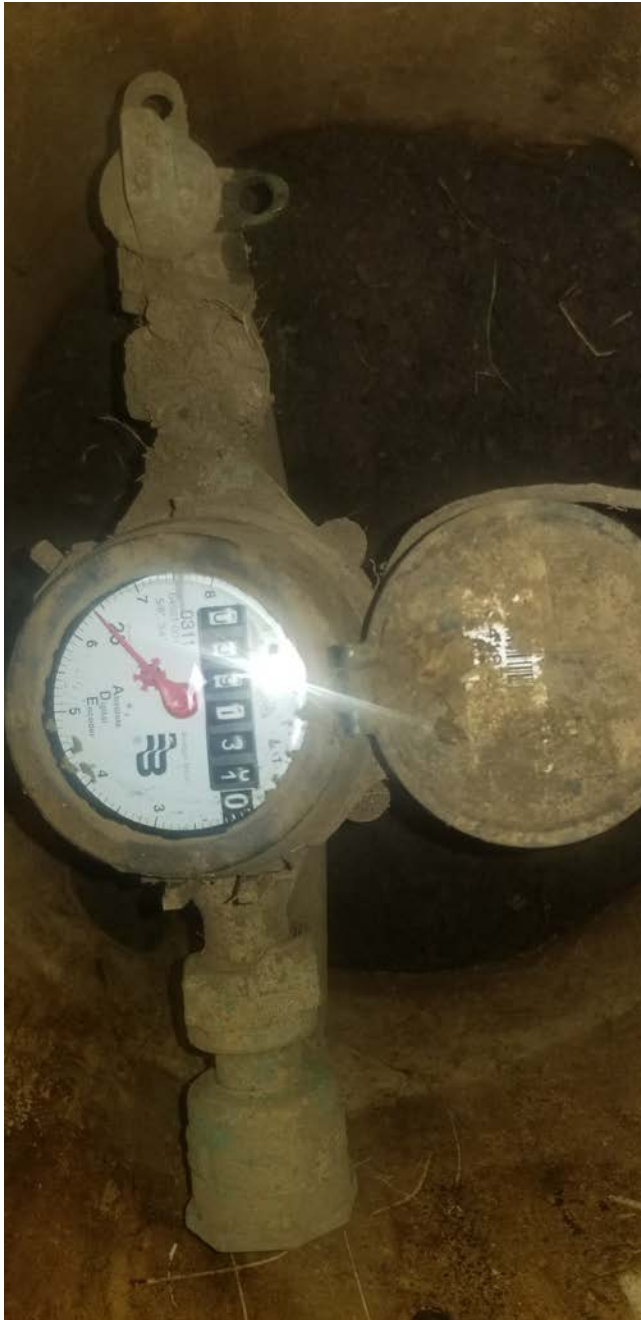
Charles Scharf new meter. Swapped out after complaints of low water pressure
