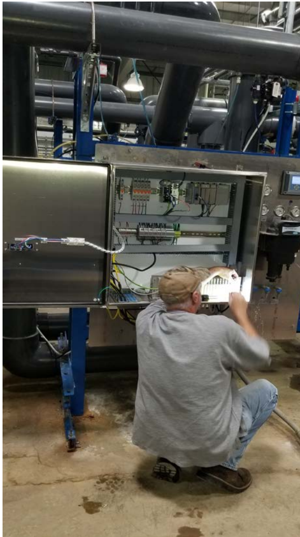
Plant staff replacing actuator card on train #2.
