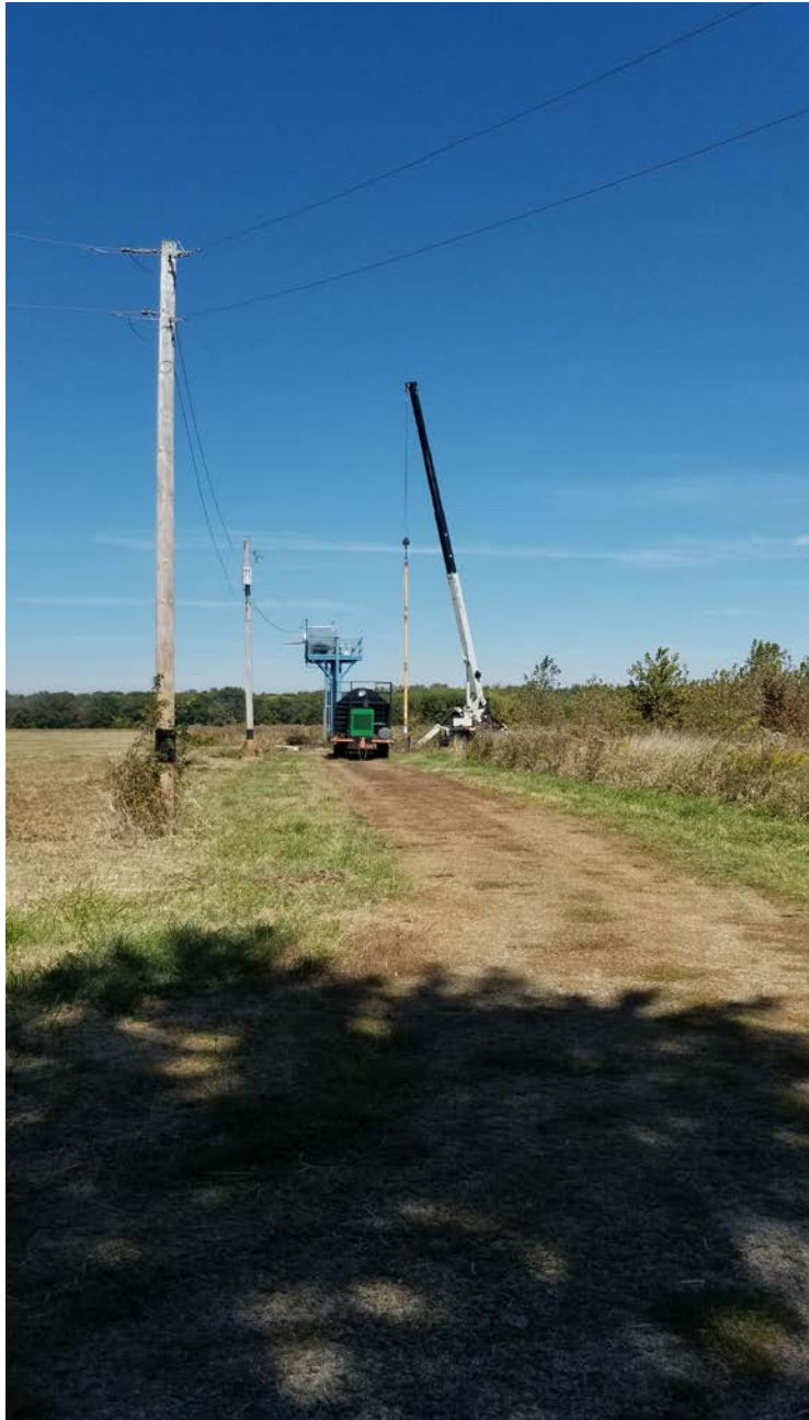
Replacing the pump and motor of well #8.
