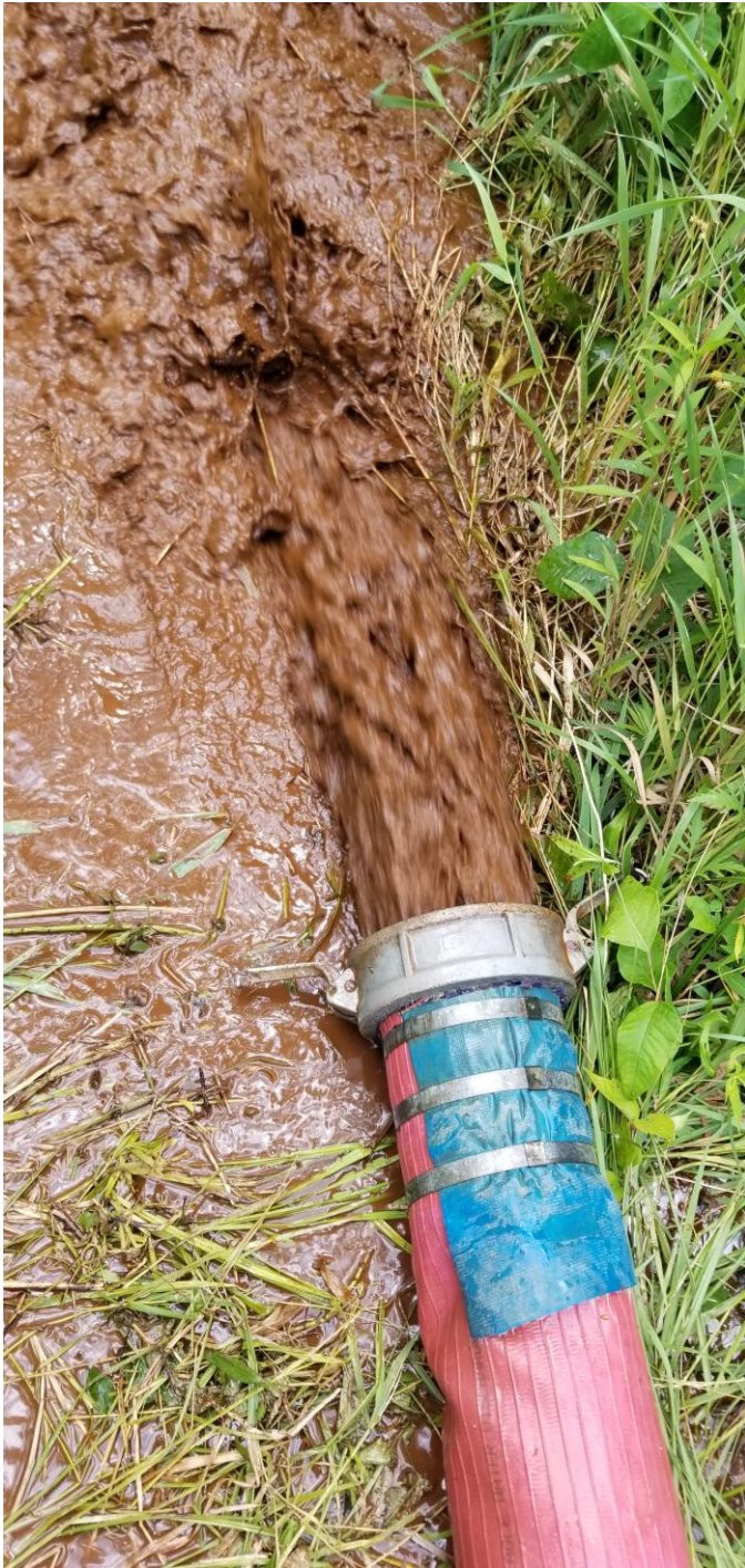
Backflushing well #10 after Brotke finished clean the well cleaning
