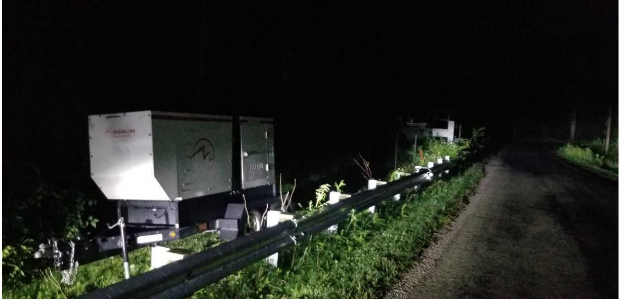
When the storms came through the booster station lost power. Lee electric brought a generator out to provide power. The generator had to be started and monitored numerous times a day.
