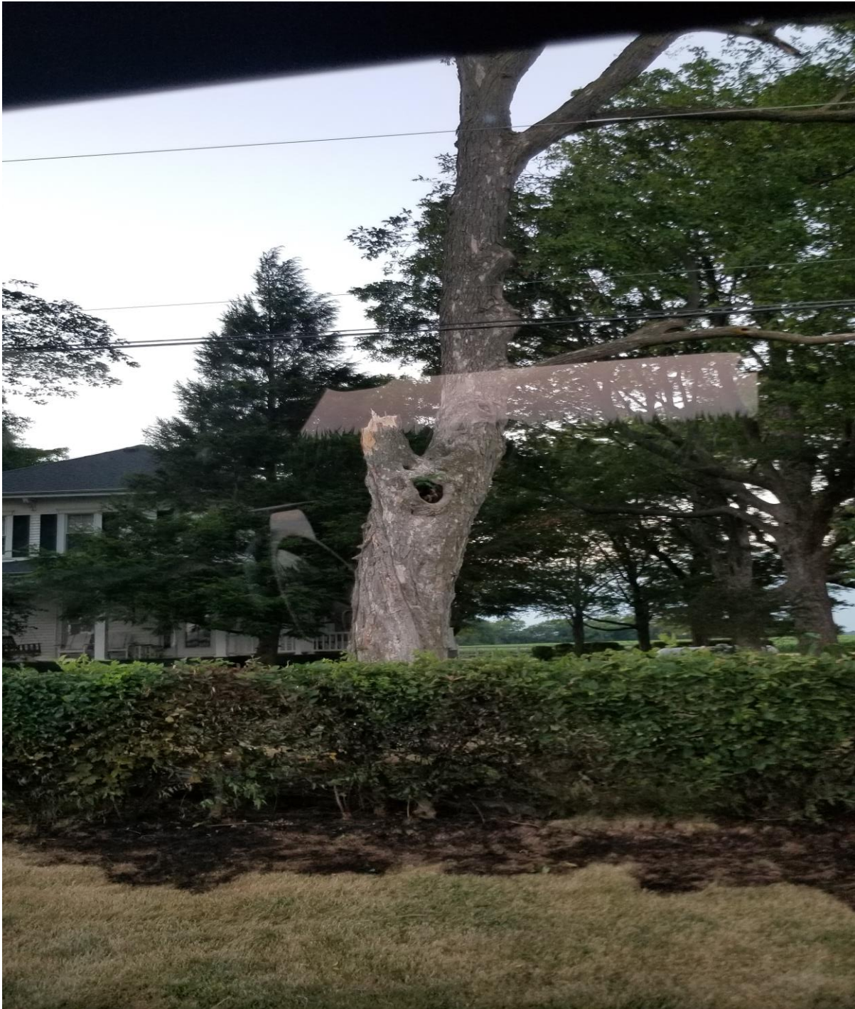
There was a downed tree limb on Buckhart that caused a power interruption.
