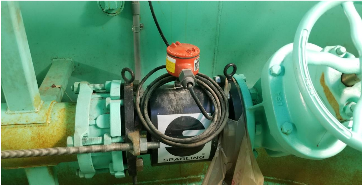
The booster station flow meter has stopped transmitting flow
