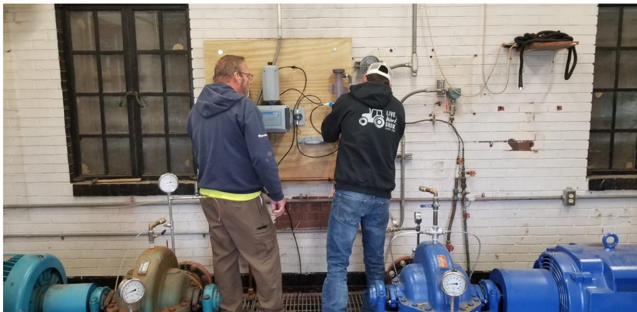
Interconnect turbidimeter has been installed and is operational
