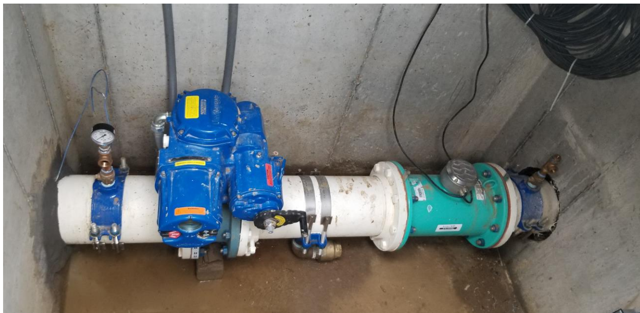
Chatham/SSWC interconnect valve has been installed.
