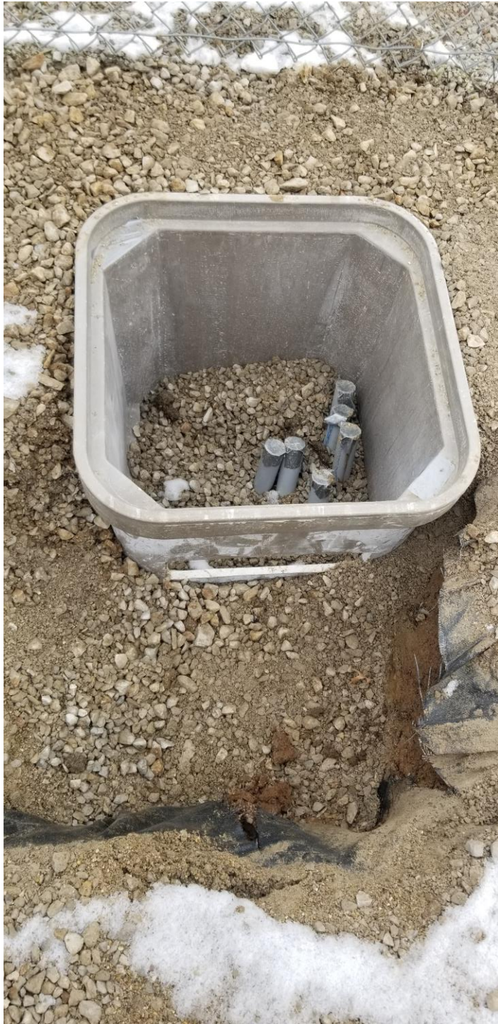
Line bores for interconnect valve control wiring and power lines
