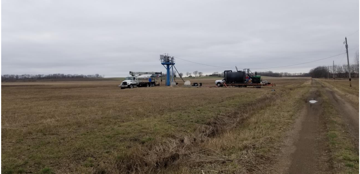
Brotke pulling well #5 before starting the clean.
