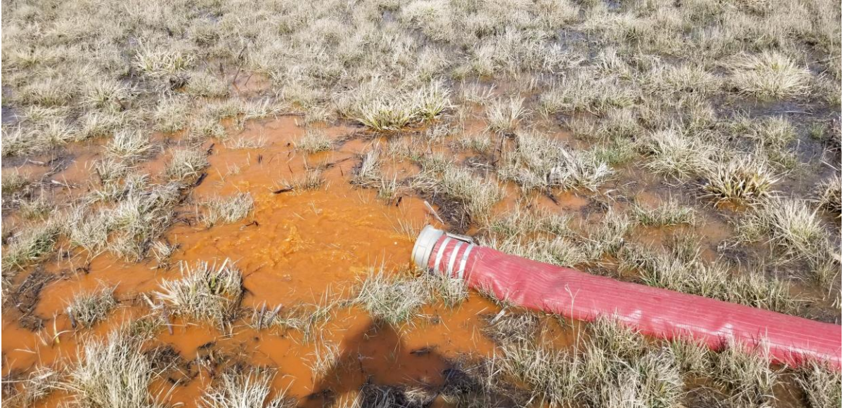
Well #7 was backflushed before being put back on line
