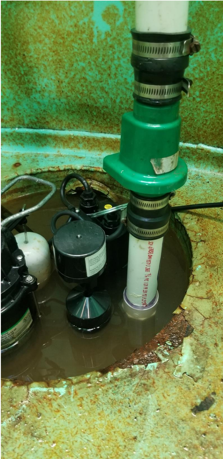
A new sump pump was installed in the New Berlin Booster station
