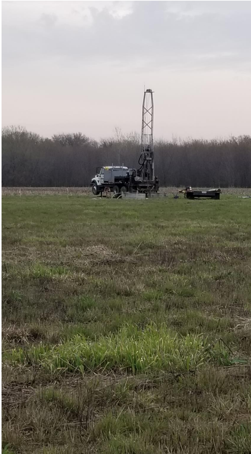
Brotke on site drilling #11 sample well.
