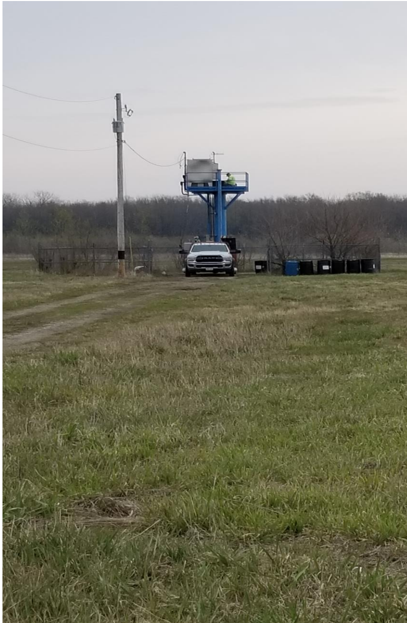
Brotke installing a new transducer well #7
