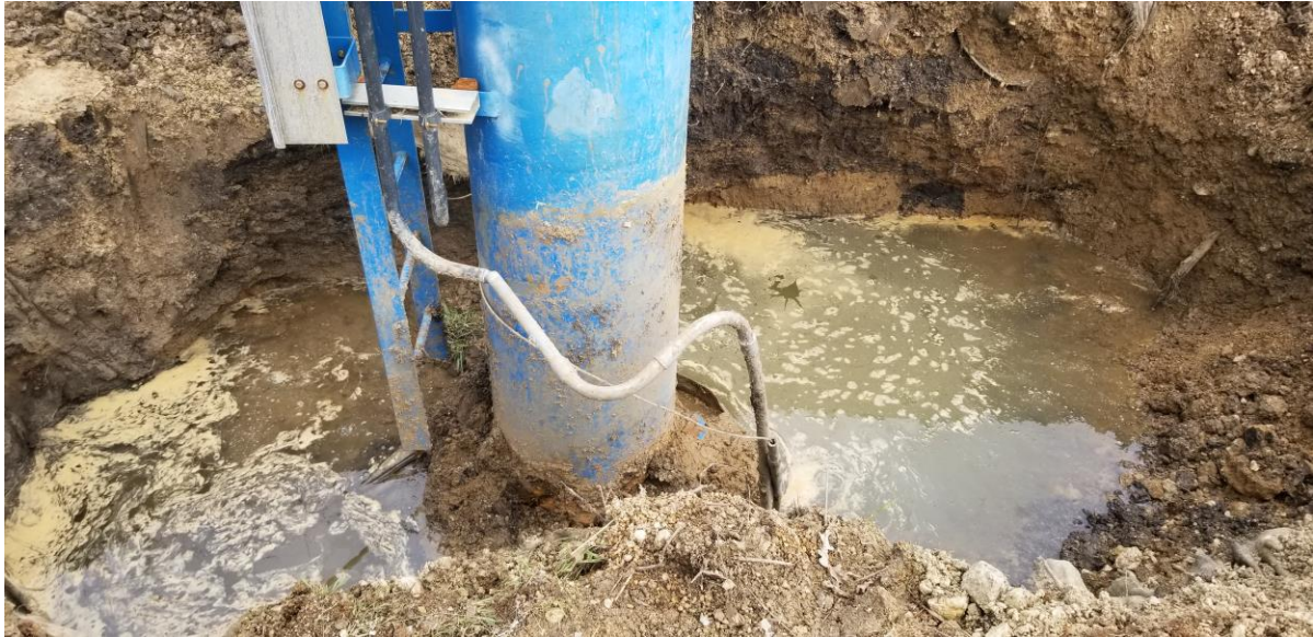
Well #3 has been partially excavated
