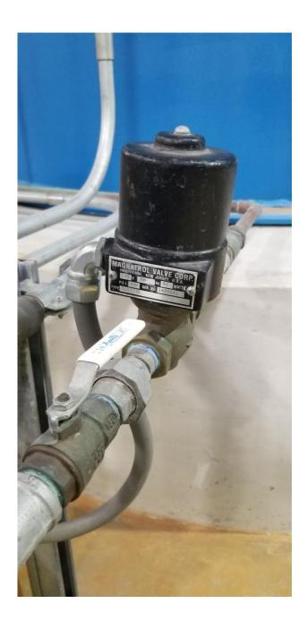
The air inlet valve on the hydropneumatics tank wasn't opening
