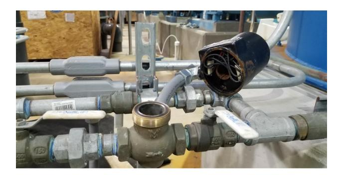
Upon inspection it was found that the interior of the valve was corroded. After disassembly the inner workings were cleaned allowing the valve to operate properly.
