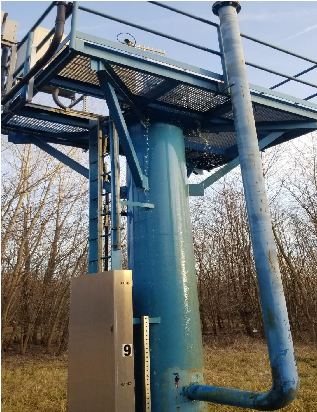
With the check valve at well #9 being bad when the plant lost power it caused the other wells to backfeed through well #9. We currently have well #9 valved out.
