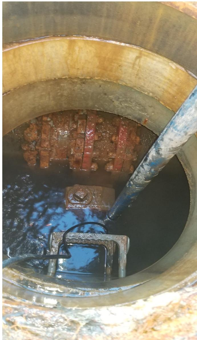
The valve pit was found to be flooded and during pump down it was found that the leak was in the pit.
