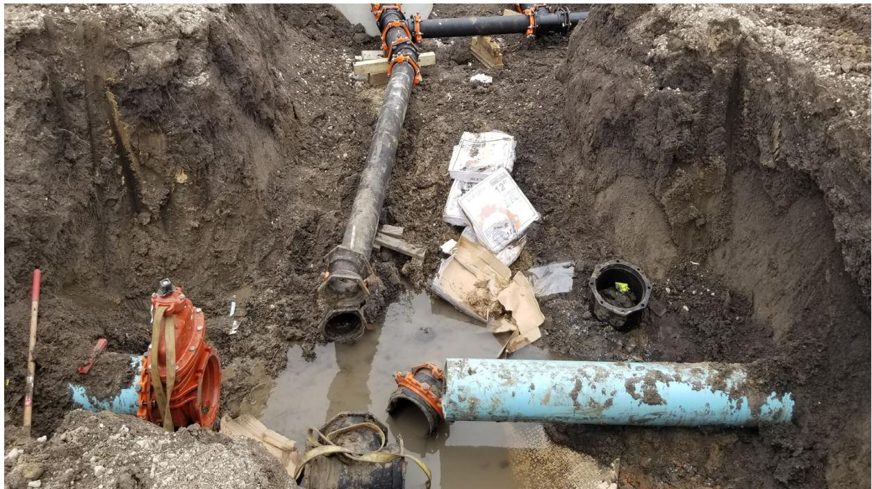
The piping for well #11 raw main has been excavated and the piping is being plumbed to tie well #11 into the rest of the wells.
