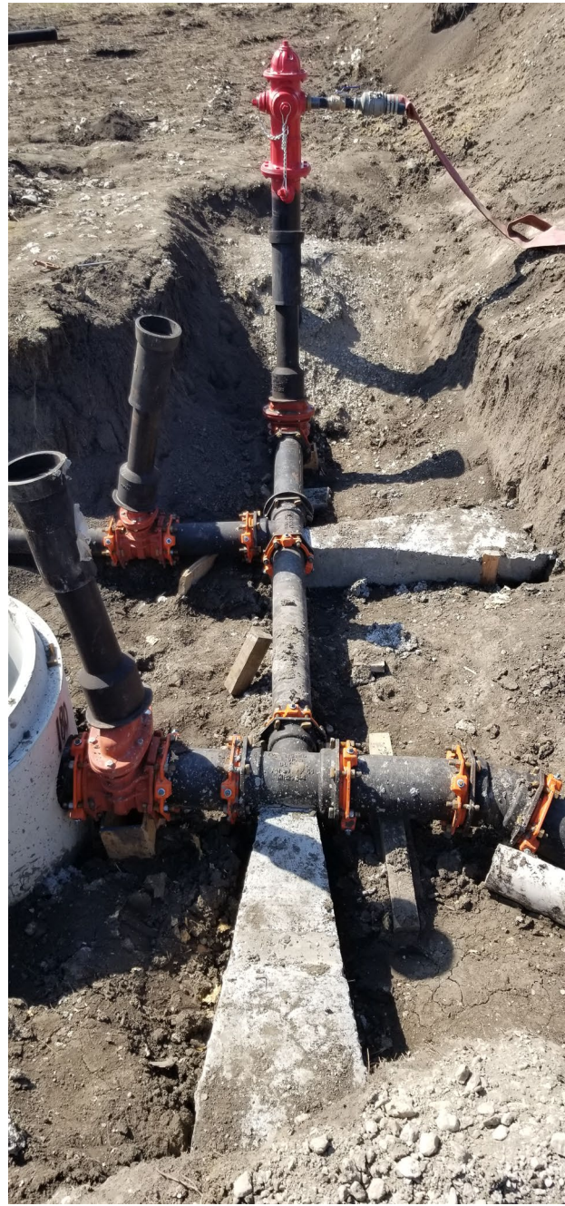
Brotke poured thrust blocks for the well #11 raw water distribution lines
