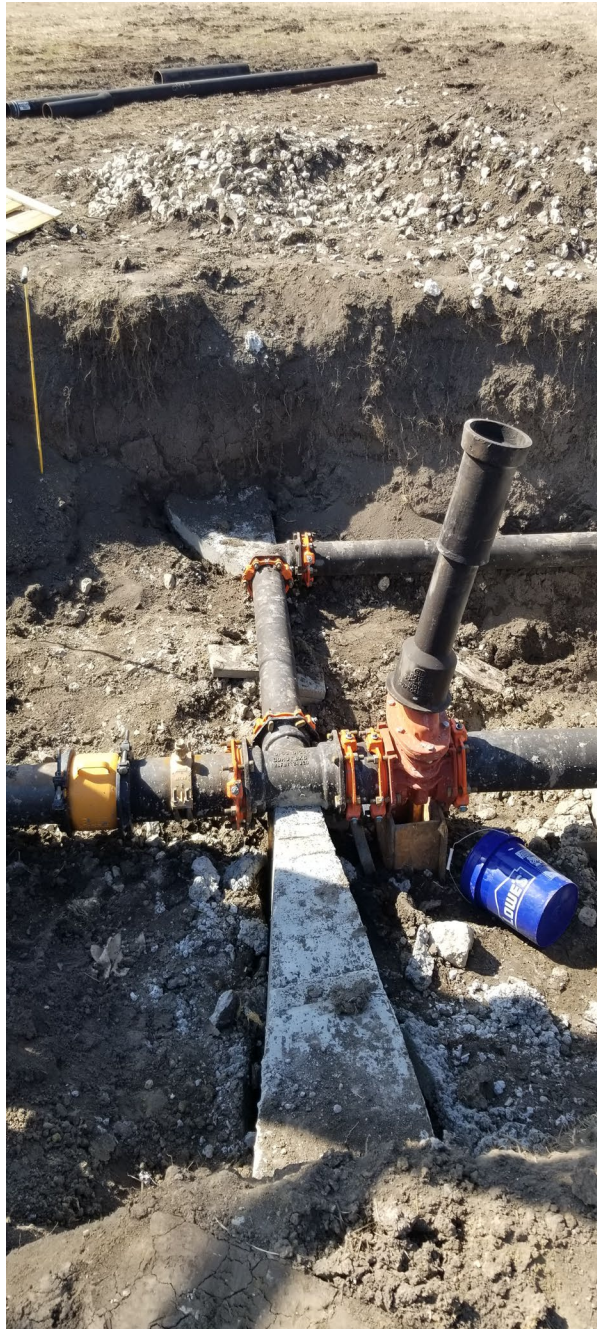
Brotke poured thrust blocks for the well #11 raw water distribution lines
