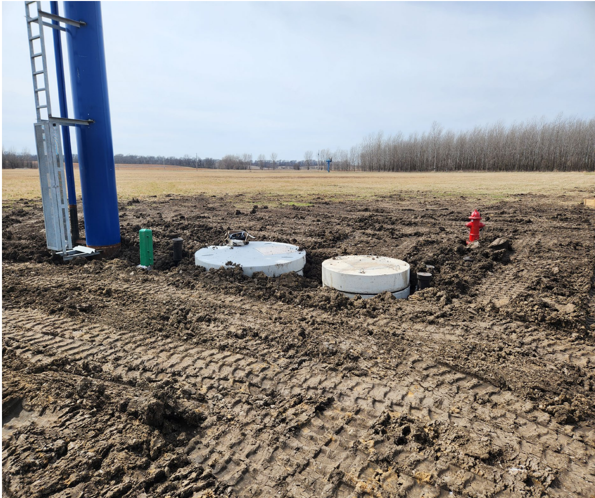
Well #11 construction site has been backfilled and rough graded.
