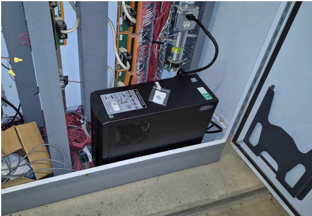
New APC battery backup for BOP.
