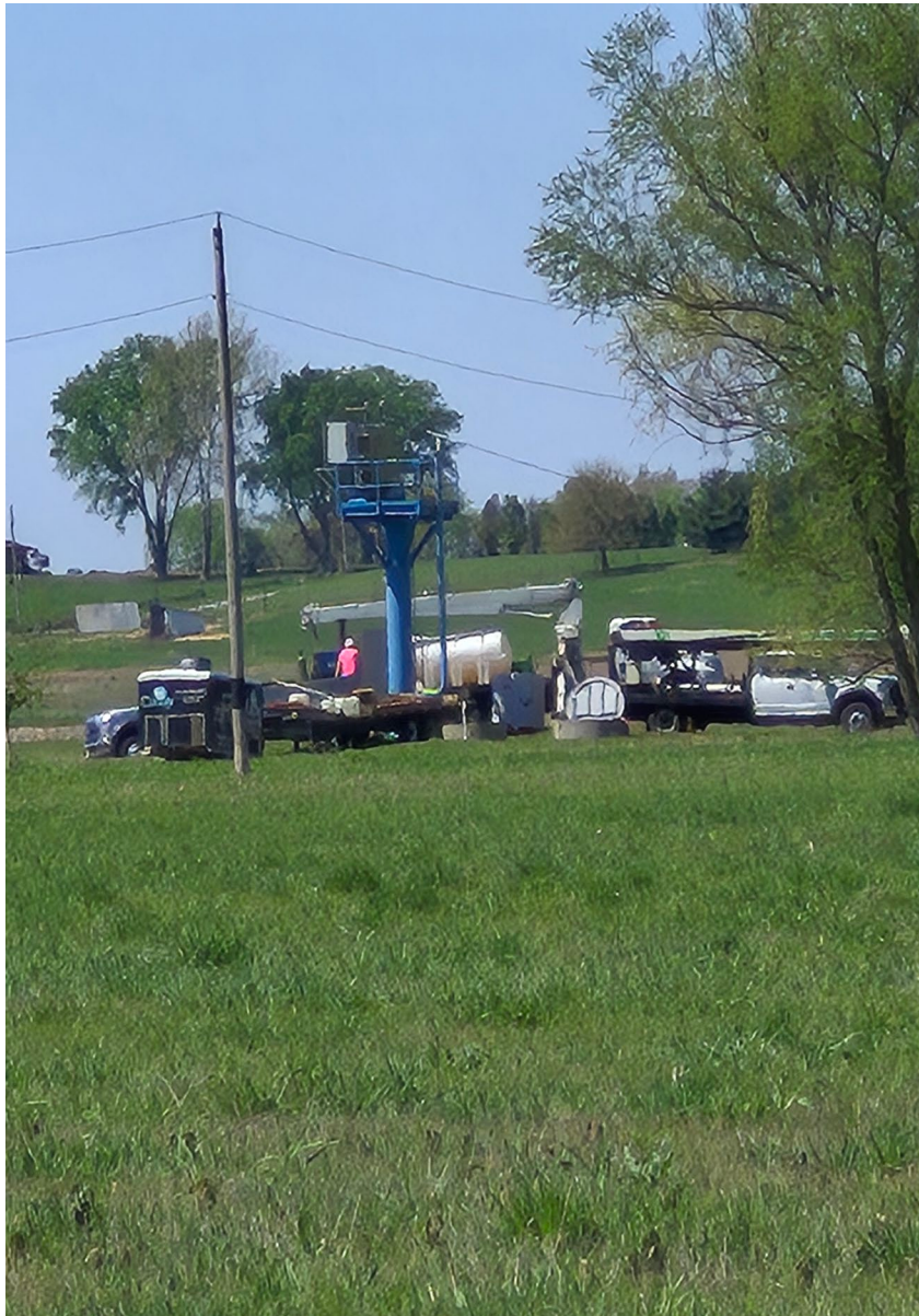
Cahoy was on site for well cleanings. This is Cahoy at well 5
