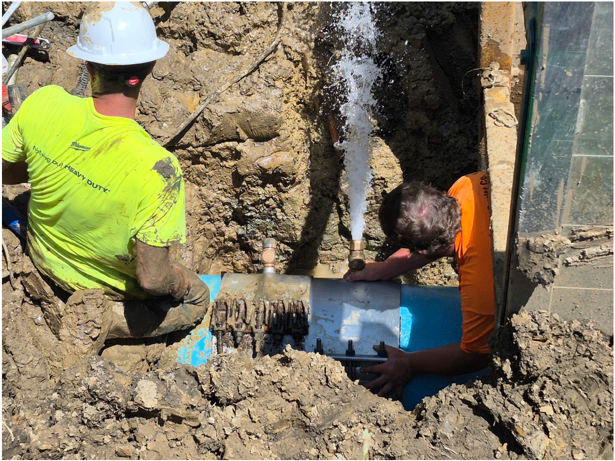
EL Pruitt installing a repair clamp with a service saddle
