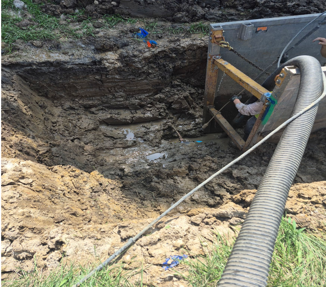
EL Pruitt excavating our water main on Cardinal Hill Rd. Staff received a call from the county about a leak
